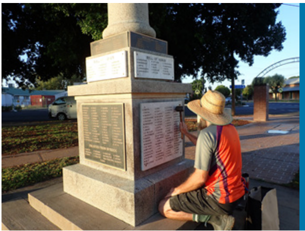
PHOTO: RGCRT Monumental-Heritage team member completing specialised traditional lead lettering work on the Bourke War Memorial, for Bourke Shire Council.
