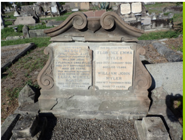
PHOTO: Again as a part of our WW1 unofficial war graves project, we worked with the Friends of Rookwood to repair and conserve Rookwood's WW1 nurses graves. This included the reinstallation of the Bessie Florence Myler monument, which had been lying face-down for decades. Reinstallation and repair of this gravestone is an important mark of respect for the self-sacrifice of this Australian Imperial Forces nurse who died of tuberculosis shortly after her overseas service.
