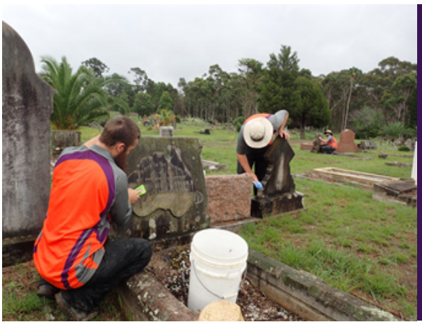
PHOTO: The RGCRT Monumental-Heritage team completing maintenance work on WW1 graves, as a part of our WW1 unofficial war graves project. Works included re-tapping lead lettering, re-attaching fallen inscription plaques, re-installing fallen monuments, removing overgrowth, and hand-cleaning inscriptions.
